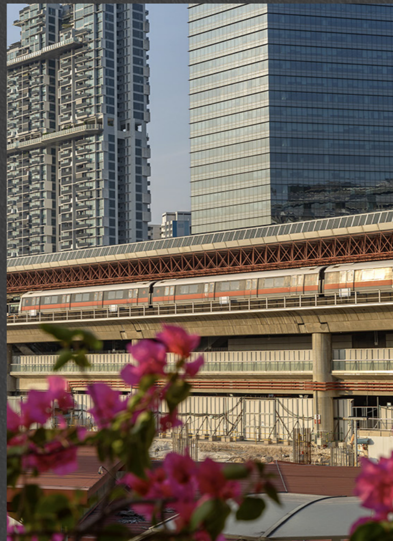
Jurong East MRT Interchange
