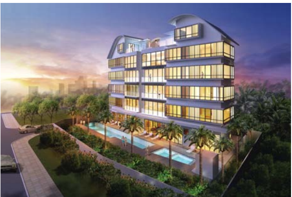
833 MB Residences (Construction in progress)
