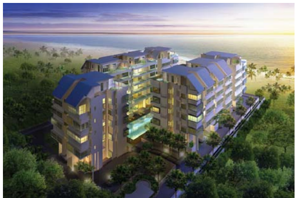
Coastal Breeze Residences (Construction in progress)
