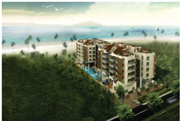
Coastal View Residences (Completed)
